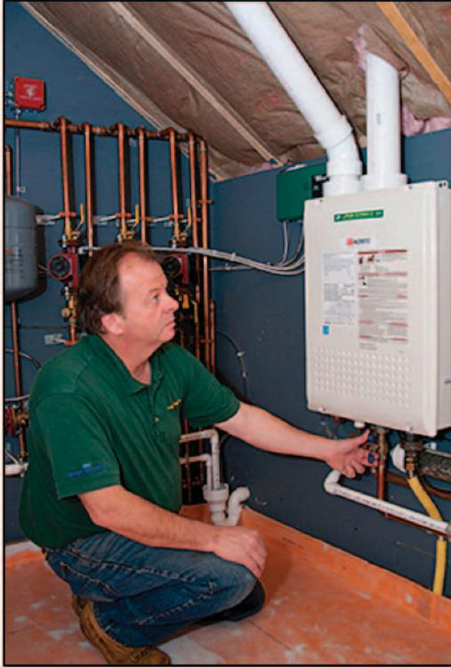
The NRC83-DV can be vented with three-inch or four-inch Schedule 40 and 80 PVC or CPVC pipe, which is less expensive and quicker to install than the Category III Stainless Steel that must be used on conventional tankless water heaters.
